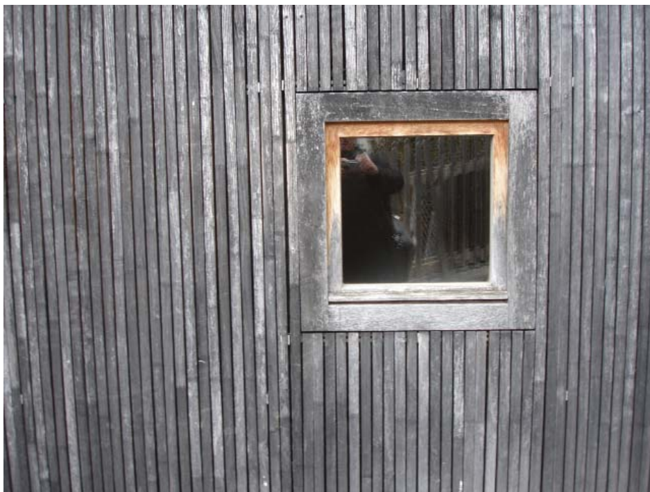
Narrow strip timber cladding without visible face fixings: Atelier Peter Zumthor, Haldenstein, Switzerland Architect Peter Zumthor 1986-86.
