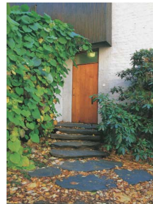
Narrow strip timber cladding without visible face fixing: Alvar Aalto House and studio, Ruuhis, Helsinki Architect: Alvar Aalto 1934-36
