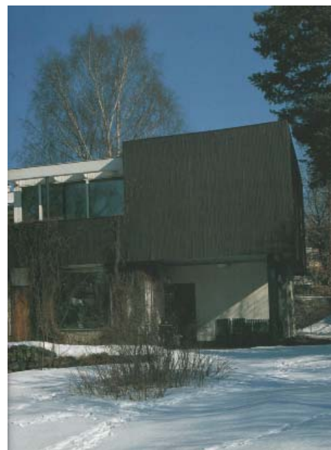
Narrow strip timber cladding without visible face fixing: Alvar Aalto House and studio, Ruuhis, Helsinki Architect: Alvar Aalto 1934-36
