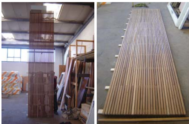
One of the façade panels ready for delivery to site to be erected onto the main structure.
