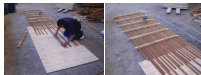
Early 1:1 detail of cladding exploring setting out and fixing of corner batten.
