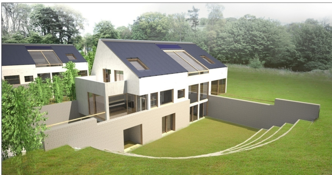
Figure 9: Z-en House South-west Façade Image
