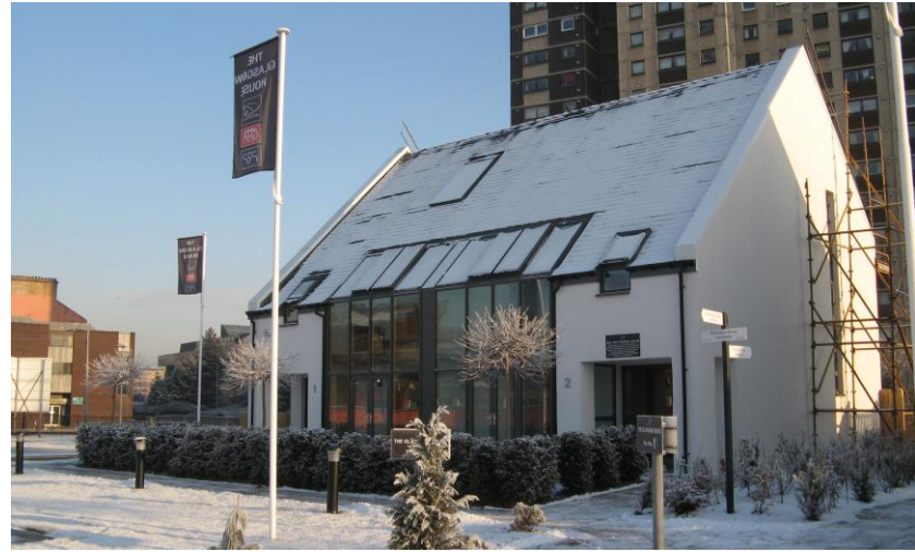
Figure 1 Glasgow House, Glasgow Housing Association
