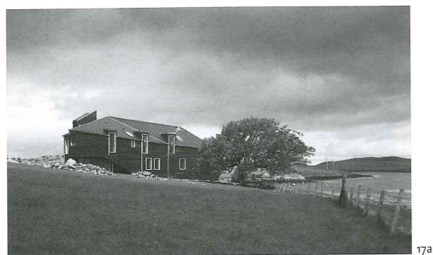
18 a-c Old and new are seen as crucial collaborators, helping to 'bed in' the new in the landscape by physically integrating it with that which was there before
