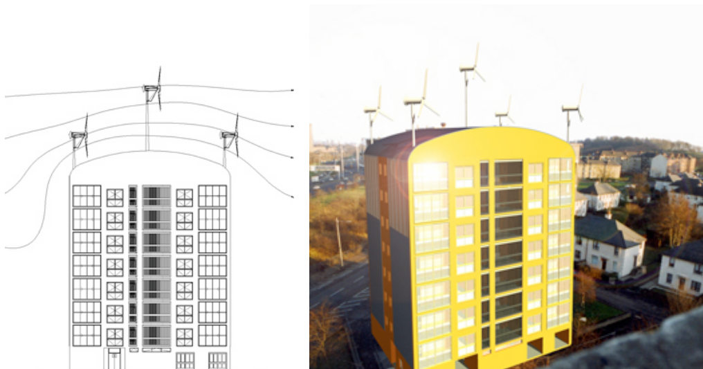
Figure 5: Curved roof forms.
